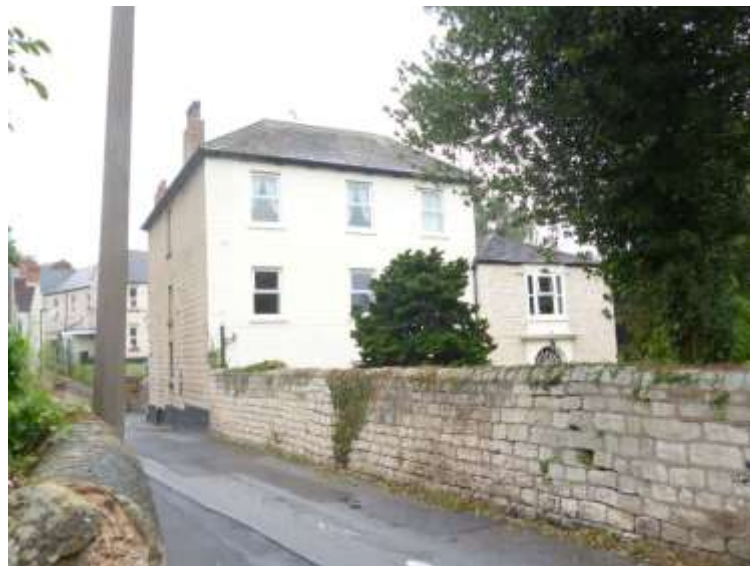
The Dale, a key unlisted building
