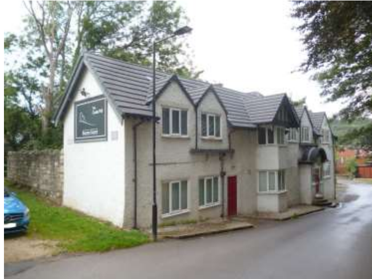
The Castle Mill Business Centre
